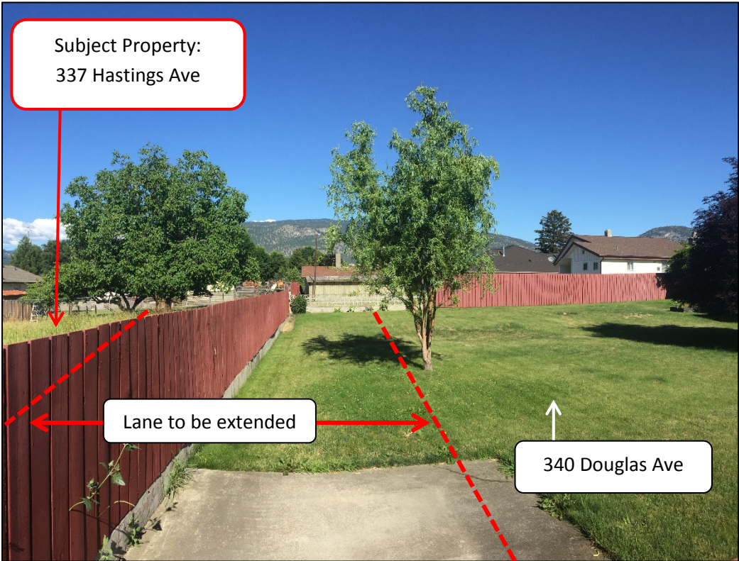
Figure 7 – Looking down the rear property line of 337 Hastings Avenue, where new lane will extend
